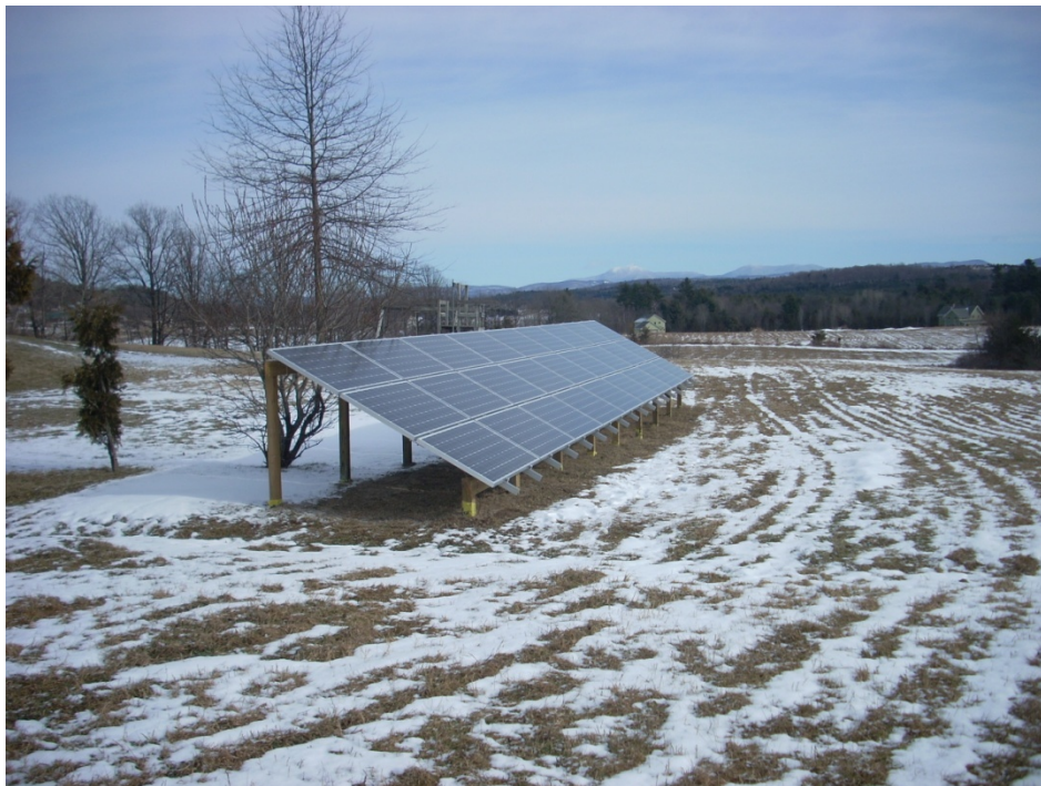
Solar Array with 30 degree pitch for maximum spring- summer-fall gains.
