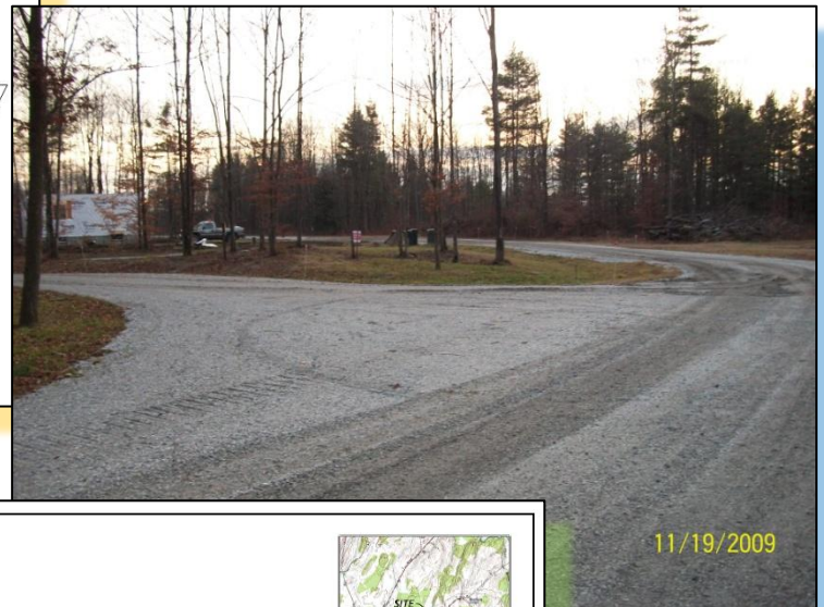
Project Road Near Completion
